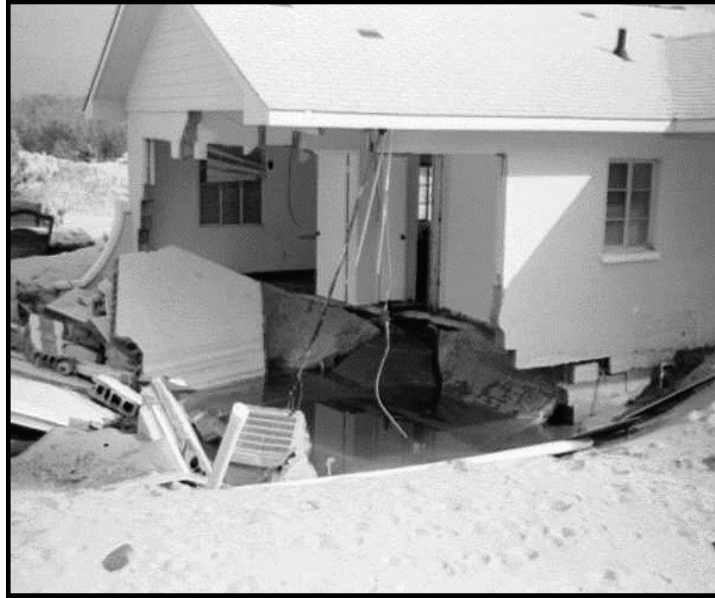
Figure 1-16. Beaches are particularly susceptible to undermining of foundations due to velocity flows.
